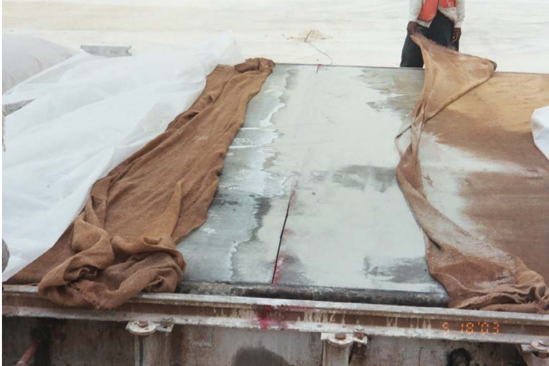
Figure 4-117 Moist Cure Method (Temporarily Removed For Saw Cutting)
