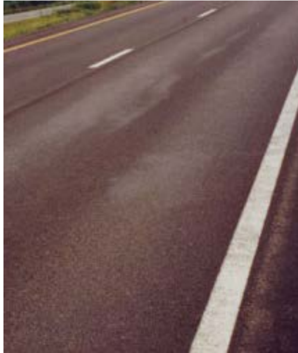
Figure 3-55 Surface Distortion
