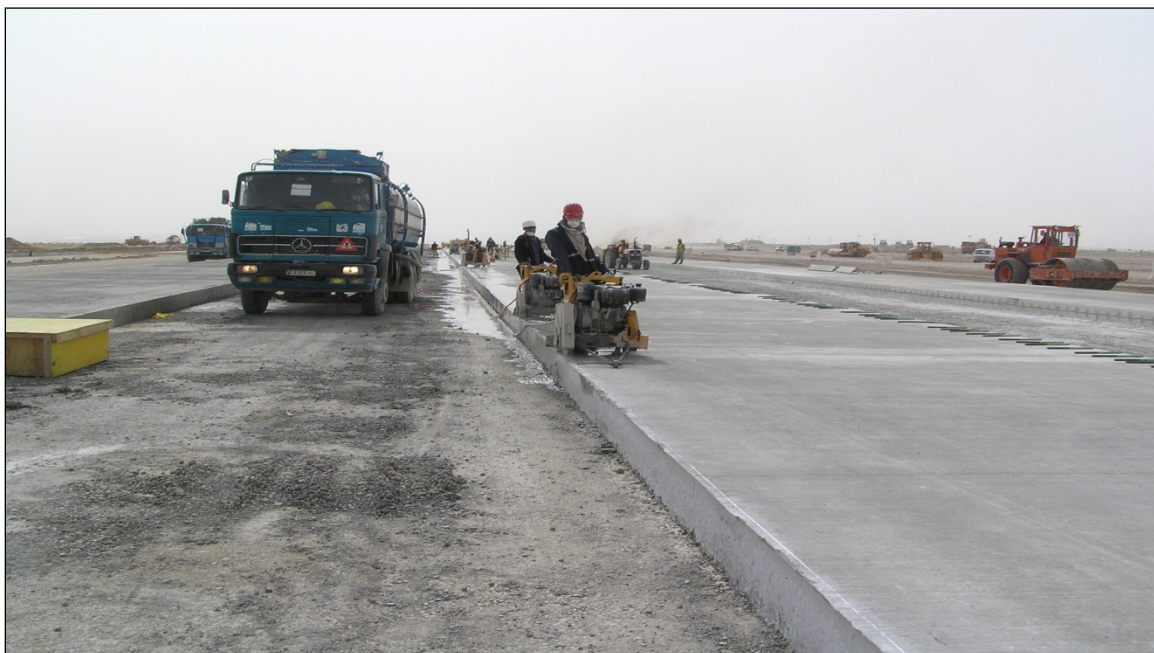
Figure 4-158 Saw Cutting Vertical Joint Face
