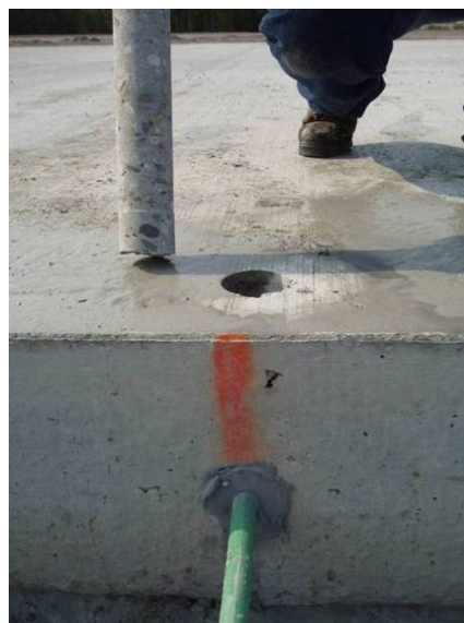
Figure 4-64 Cored Dowel to Verify the Grouting Technique
