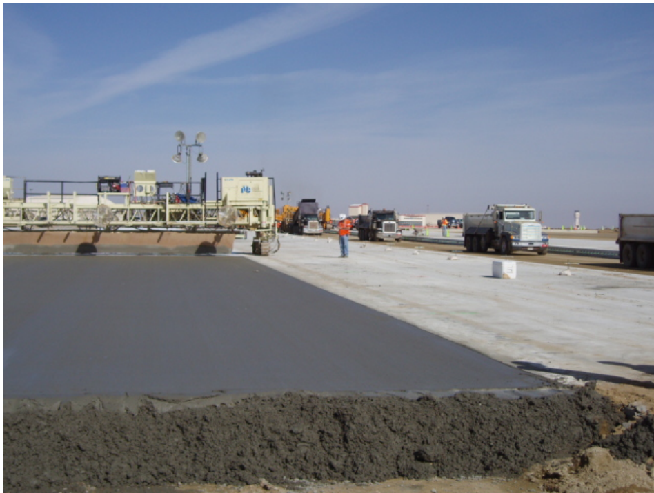
Figure 4-68 Backup of Trucks at Paving Site
