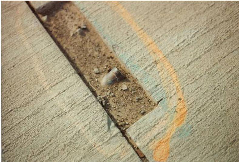
Figure 4-50 Misaligned Contract Joint Dowels
