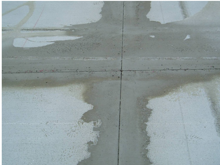
Figure 4-140 Cuttings Not Removed
