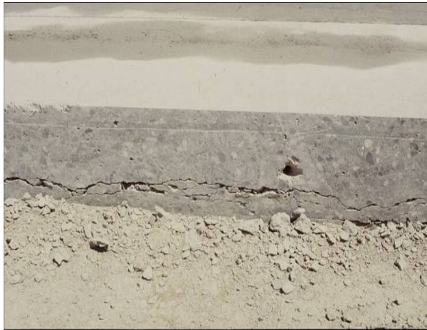
Figure 4-27 Under-breaking from Incorrect Removal Techniques
