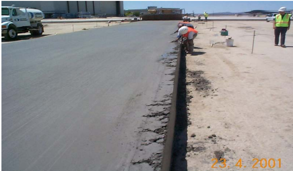
Figure 4-83 Torn and Slumped Edge on Right, Good Edge on Left. Problem is Paver Adjustment
