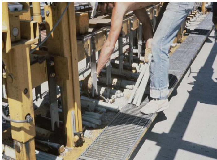
Figure 4-48 Inserting Contraction Joint Dowels – Slipform Construction
