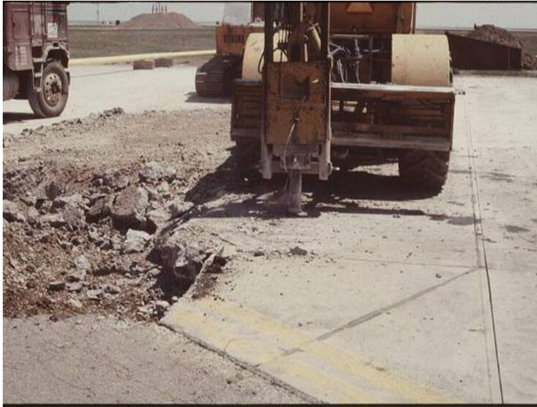
Figure 4-27 Under-breaking from Incorrect Removal Techniques
