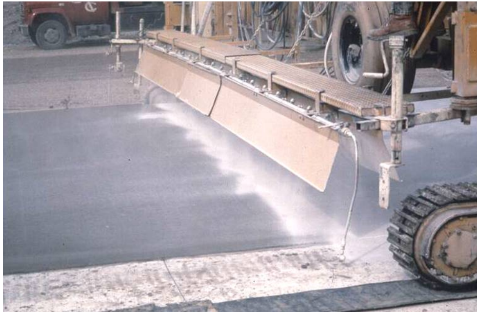
Figure 4-114 Good Application With Overlapping Spray and Windscreens
