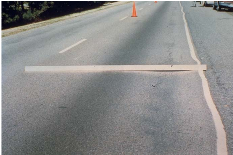
Figure 3-61 Block Cracking
