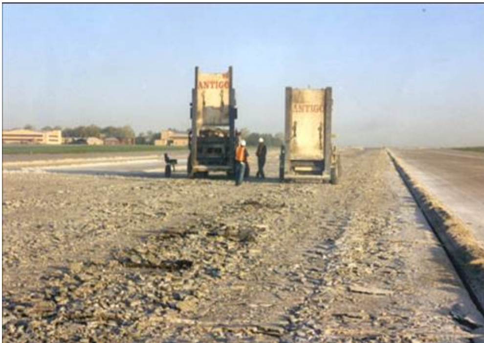
Figure 4-25 Improper removal Techniques - No Double Saw Cut
