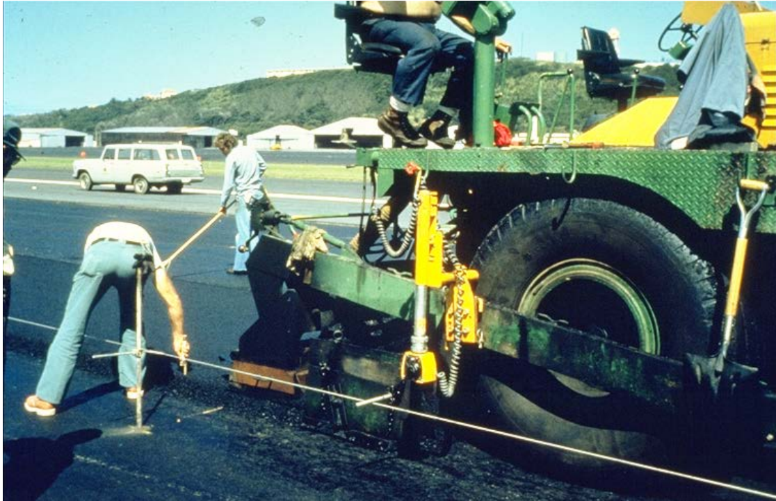
Figure 3-39 Skin Patching Should not be Allowed on the Surface
