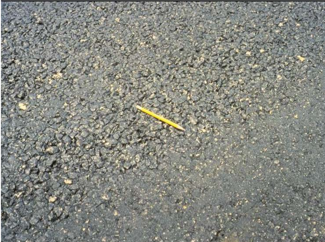
Figure 3-31 Segregation of Asphalt Mixture
