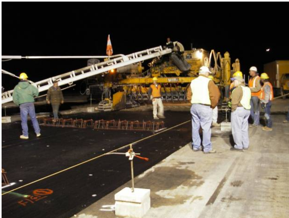
Figure 4-76 Dropping Concrete in Excess of Five Feet
