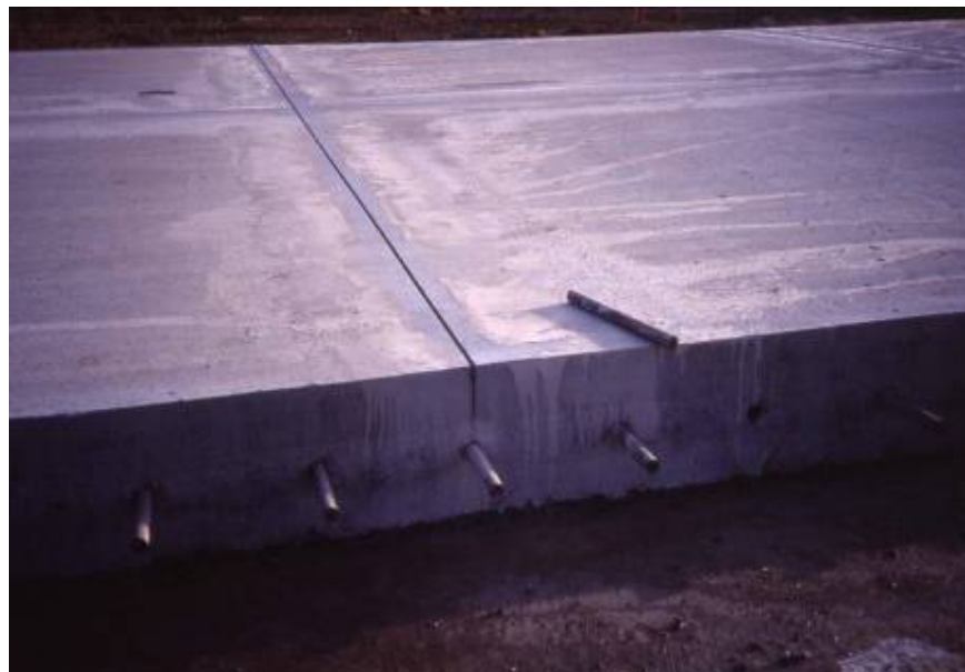
Figure 4-46 Dowel Located on a Contraction Joint.
