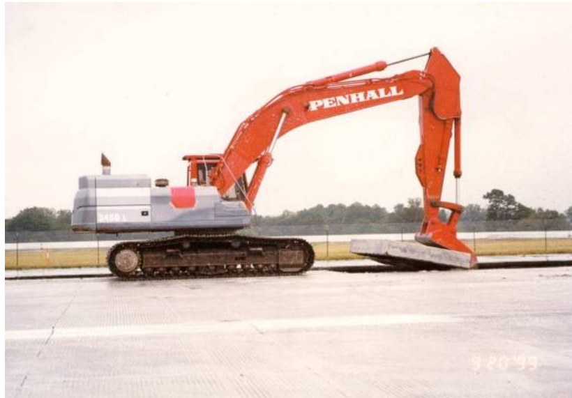
Figure 4-30 Removal of Saw-Cut Pavement Pieces
