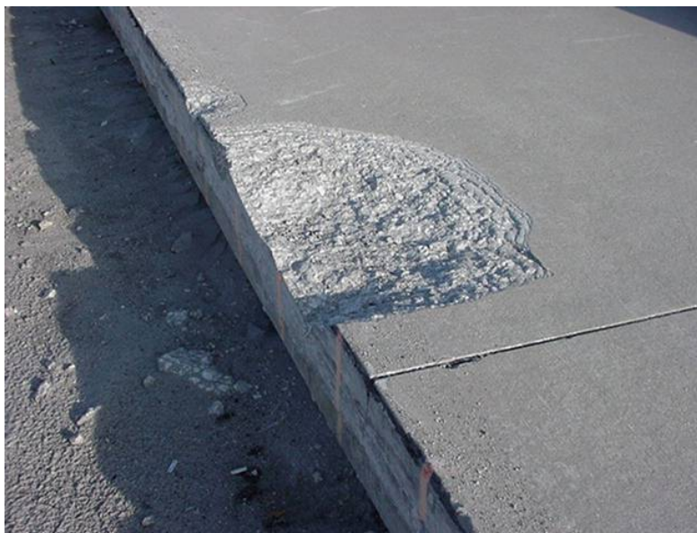
Figure 4-121 Spall Damage
