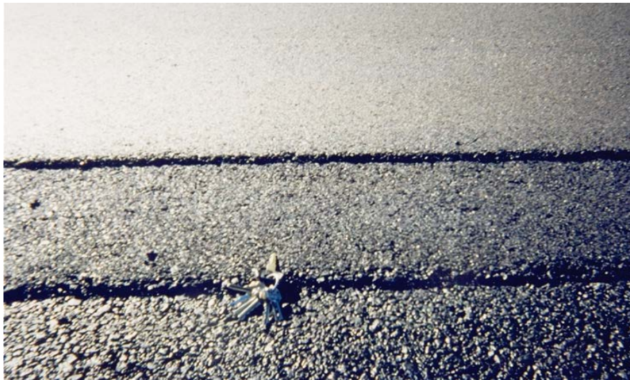
Figure 3-41 Use of Tapered Longitudinal Joint is not Desired
