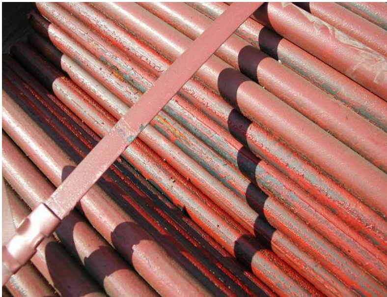
Figure 4-42 Dowels Installed on Construction Joint (Note: Not Epoxy Coating)
