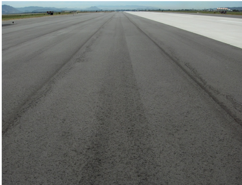
Figure 3-34 Uneven Surface after Compaction
