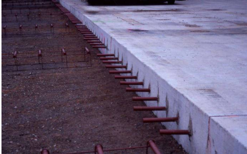
Figure 4-43 Dowel Ends not Epoxy Coated
