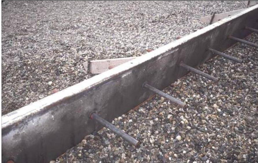
Figure 4-51 Dowels in Steel Forms
