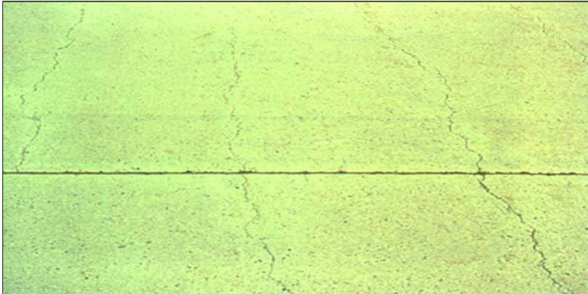
Figure 4-99 Vibrator Trails (Note Uniform Spacing Corresponding to Vibrator Spacing)
