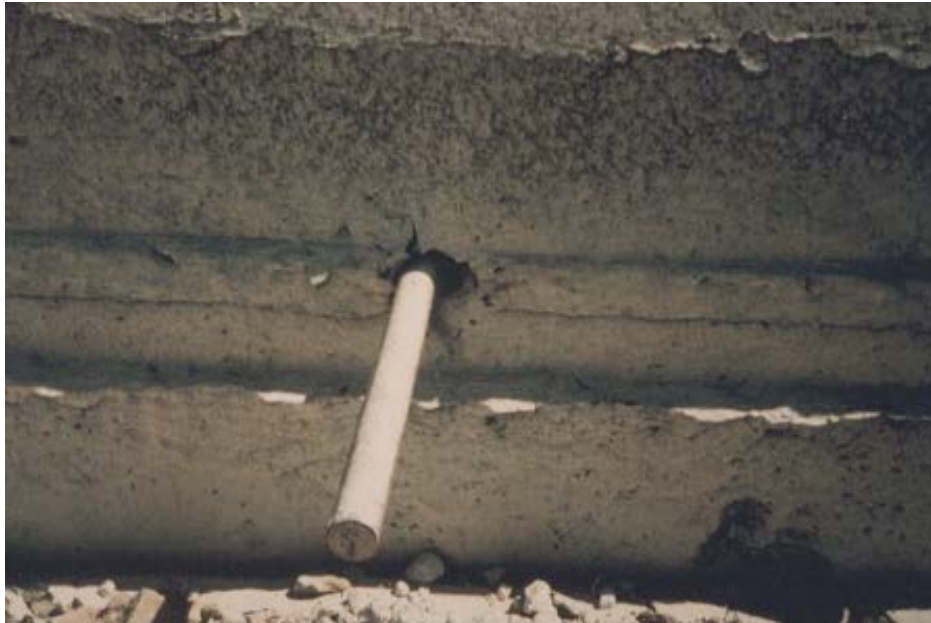
Figure 4-54 Voids around an Inserted Dowel
