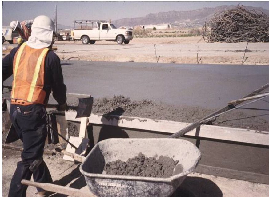
Figure 4-86 Unacceptable Repair of Edge Slump. No Full-Depth Face Support, So Vibration is Impossible
