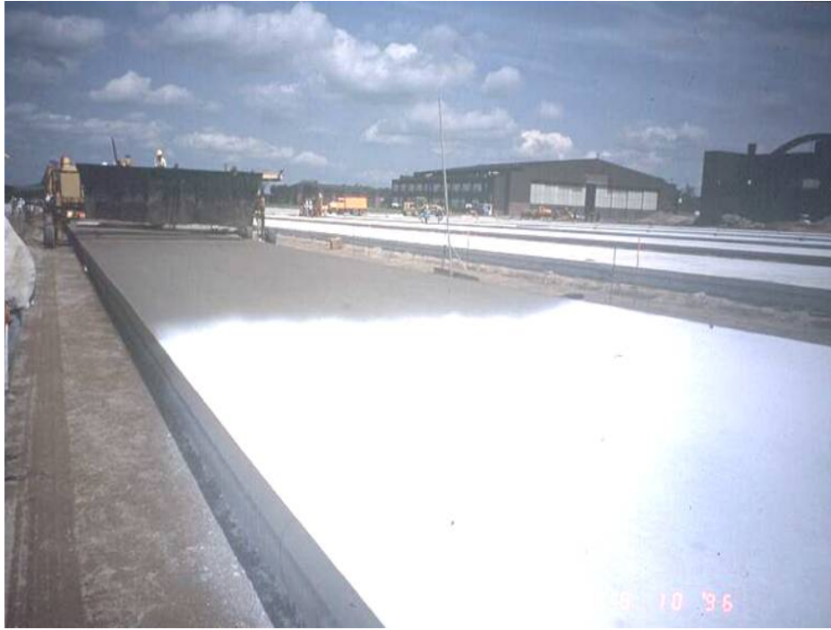
Figure 4-114 Good Application With Overlapping Spray and Windscreens
