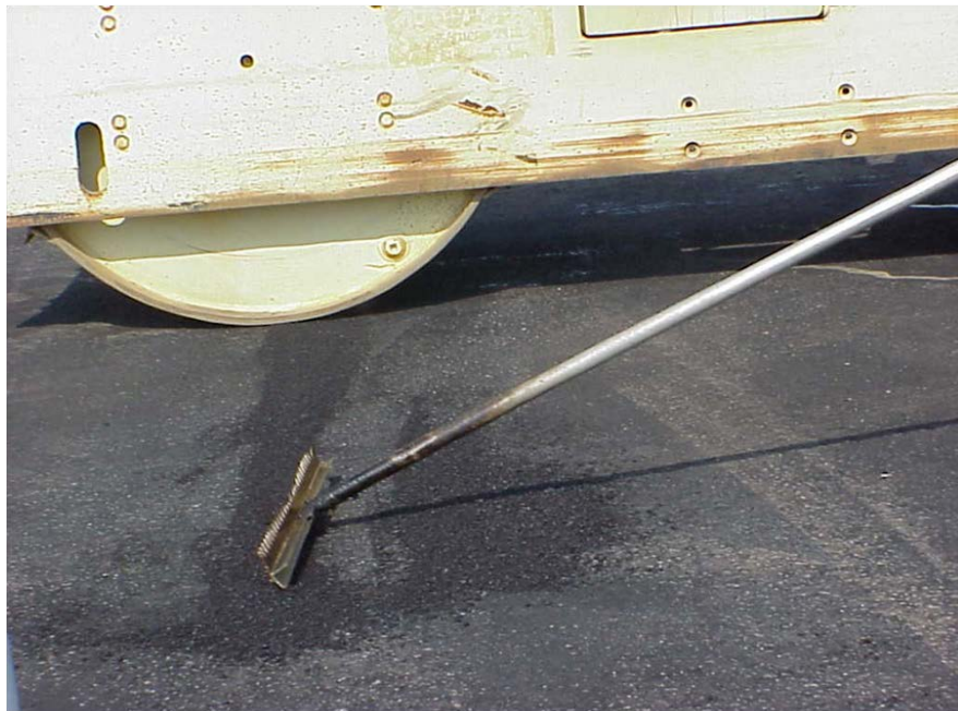
Figure 3-39 Skin Patching Should not be Allowed on the Surface
