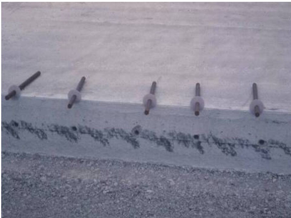
Figure 4-62 Dowels with Grout Retention Rings. Note: Excessive Spalling from Drilling in Center Drill Hole
