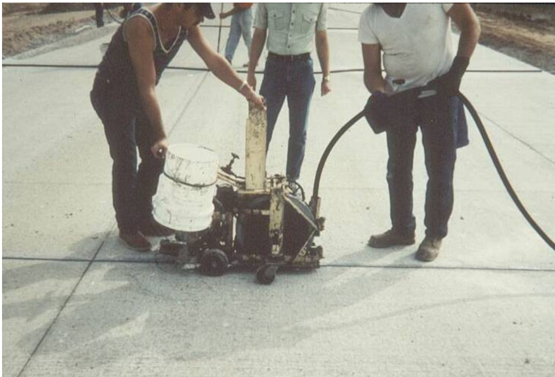
Figure 4-152 Installation Of Preformed Joint Seal – Minimal Stretch
