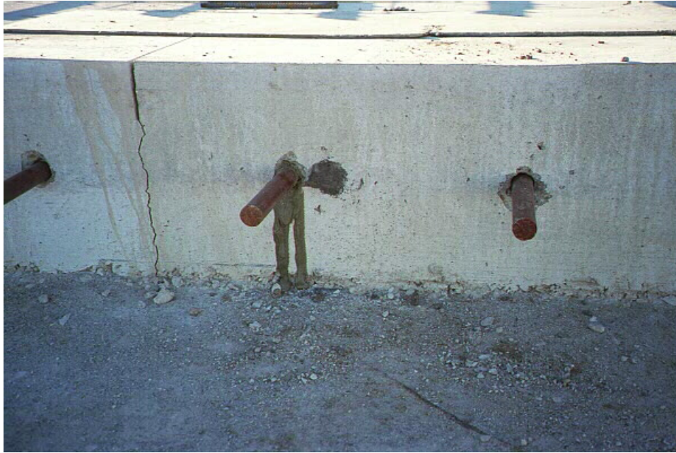
Figure 4-61 Grout Leakage with No Retention Ring
