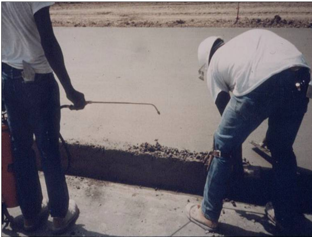
Figure 4-161 Over Finishing Edge of Pilot Lane
