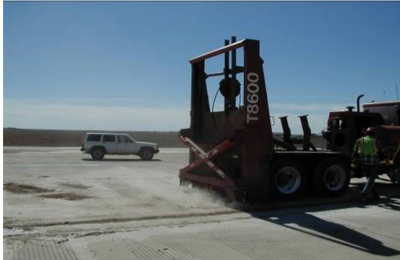
Figure 4-29 Demolition With No Protection of Adjacent Concrete
