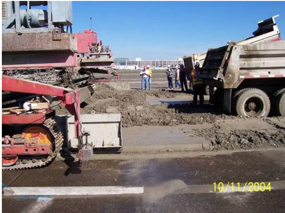
Figure 4-77 Backing Trucks Down Paving Lane
