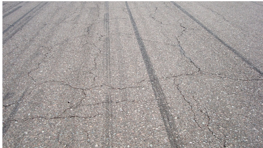
Figure 3-61 Block Cracking
