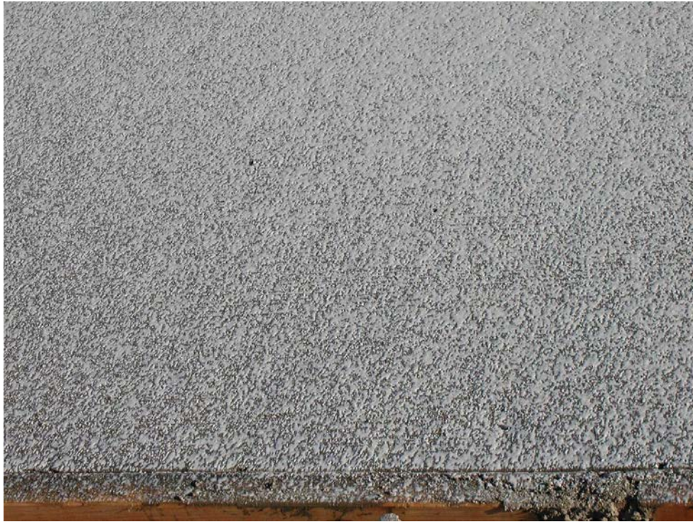
Figure 4-119 Excessive Rain Damage
