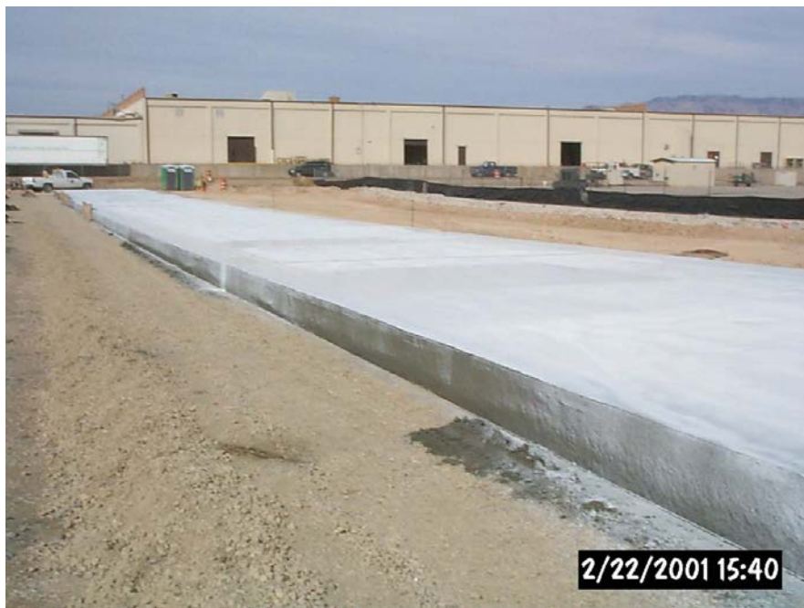
Figure 4-116 Poor Application of Curing Compound Vertical Joint
