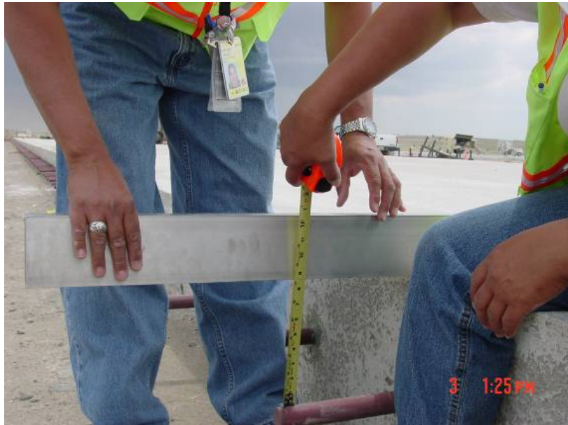
Figure 4-67 Checking Dowel for Vertical Alignment
