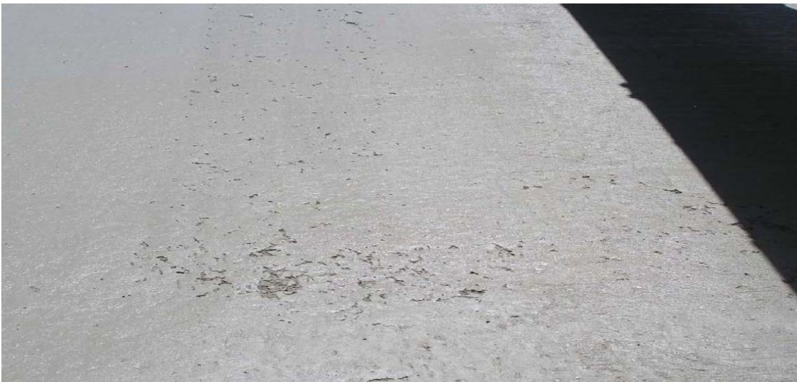
Figure 4-92 Torn Surface (Mix Was Deficient in #4 and #8 Aggregate Sizes)
