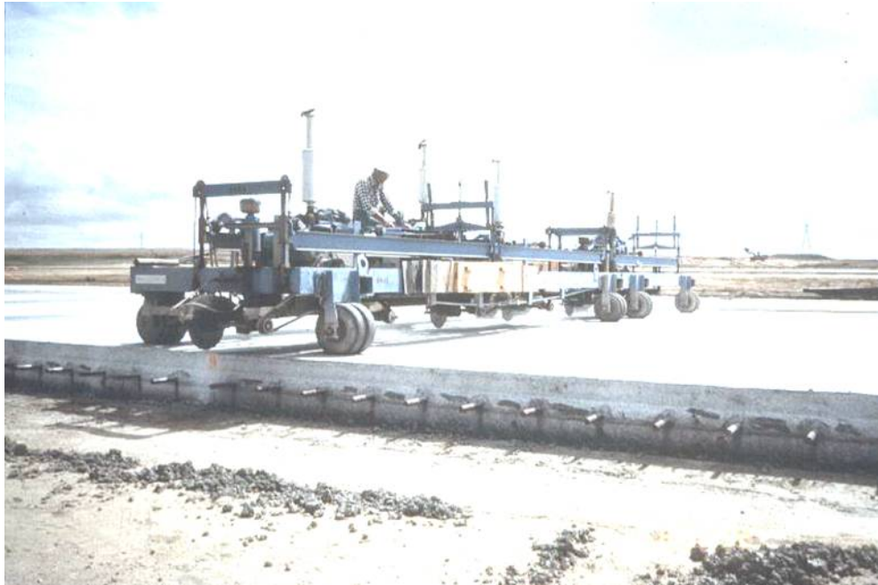
Figure 4-116 Poor Application of Curing Compound Vertical Joint
