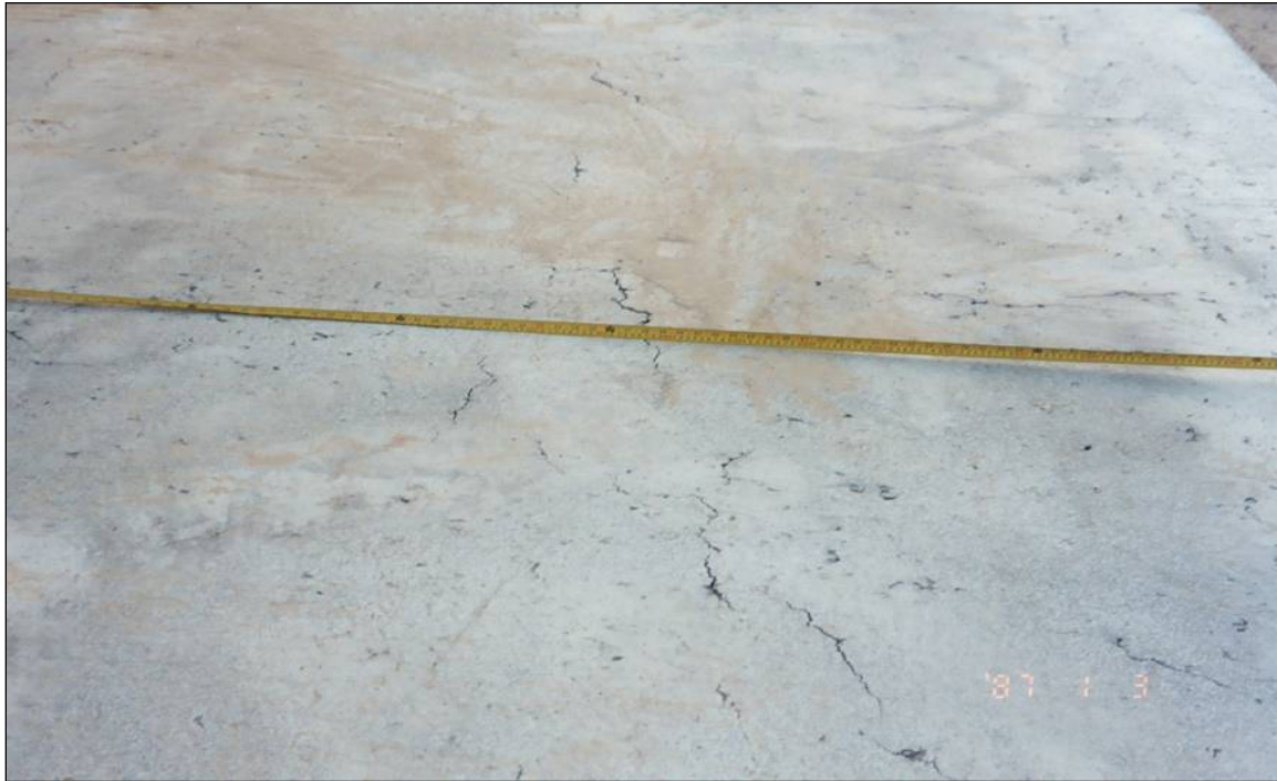
Figure 4-159 Plastic Shrinkage Cracking
