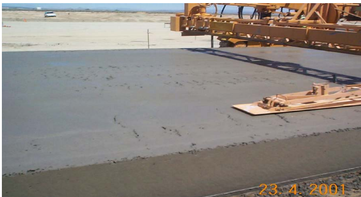
Figure 4-81 Poor Consolidation on Horizontal Surface of Slab
