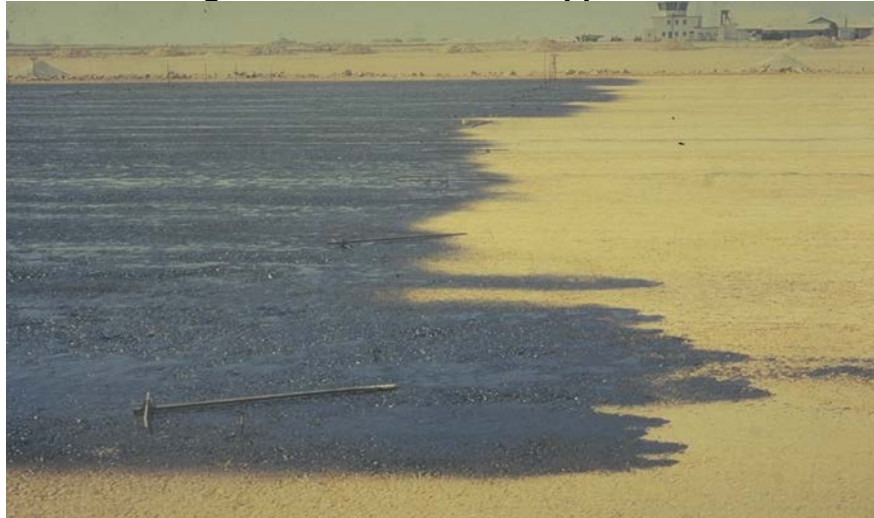
Figure 3-25 Prime Coat Application
