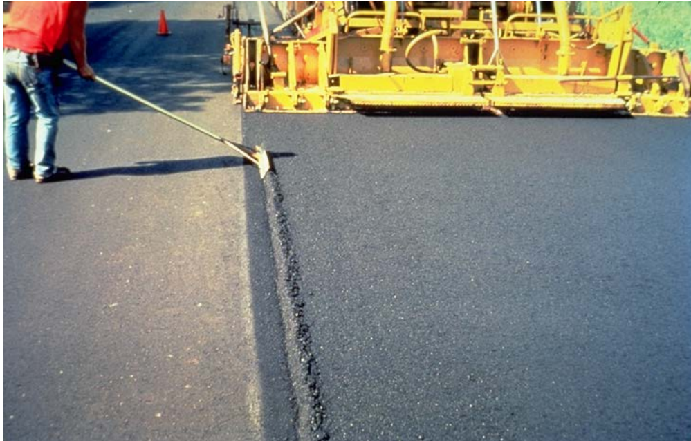
Figure 3-35 Proper way to Rake Joint
