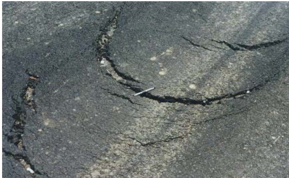
Figure 3-58 Slippage of Asphalt Mixture over Underlying Layer
