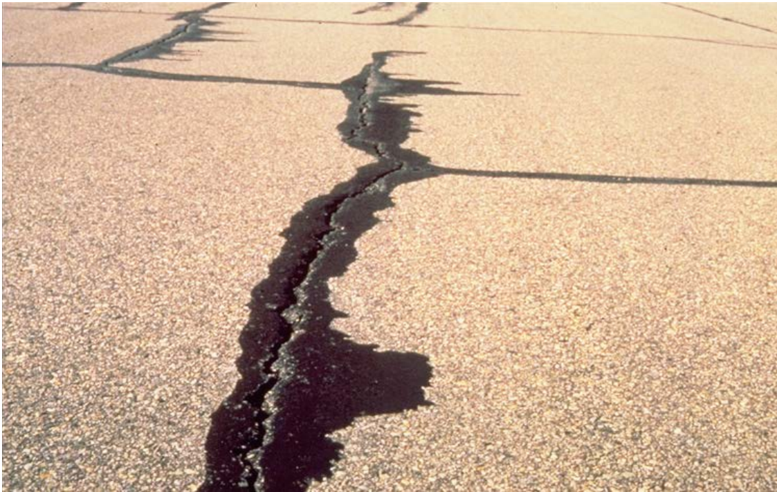
Figure 3-19 Excess Sealant
