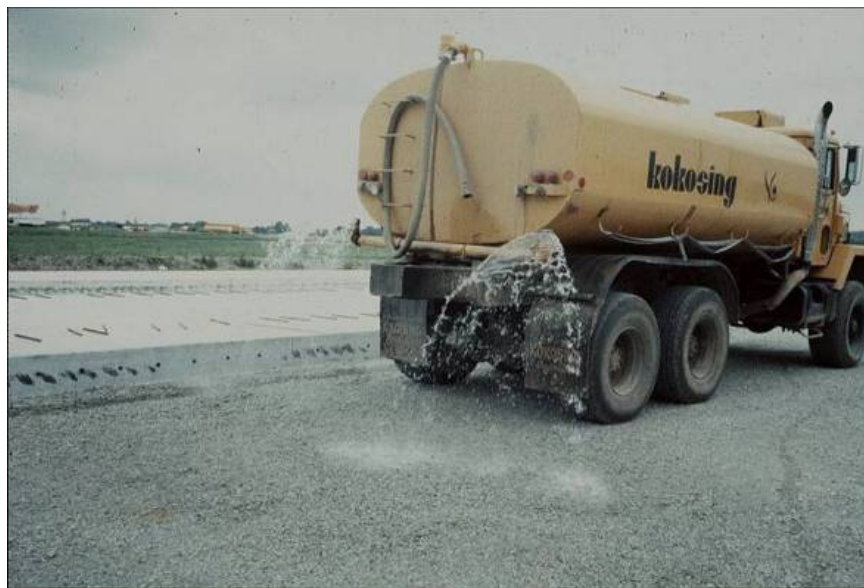
Figure 4-19 Dampening the Base Course
