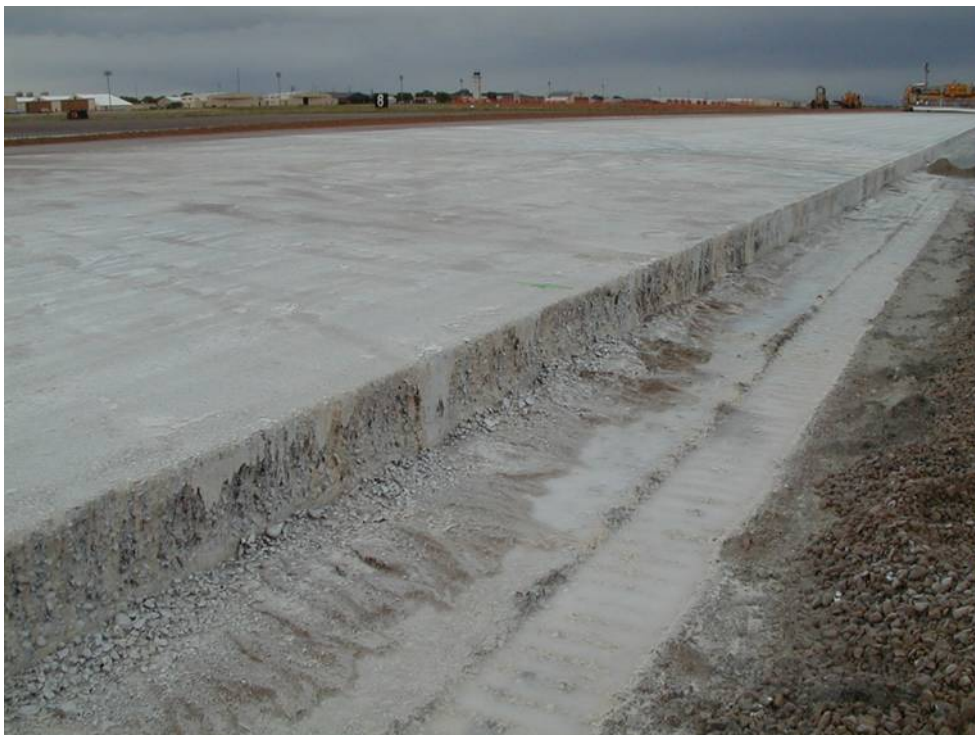
Figure 4-119 Excessive Rain Damage
