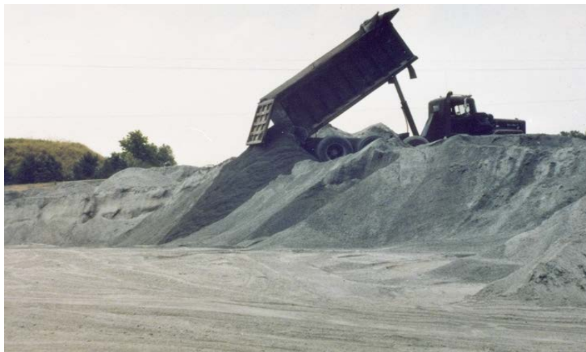
Figure 3-6 Improper Addition of Material to a Stockpile
