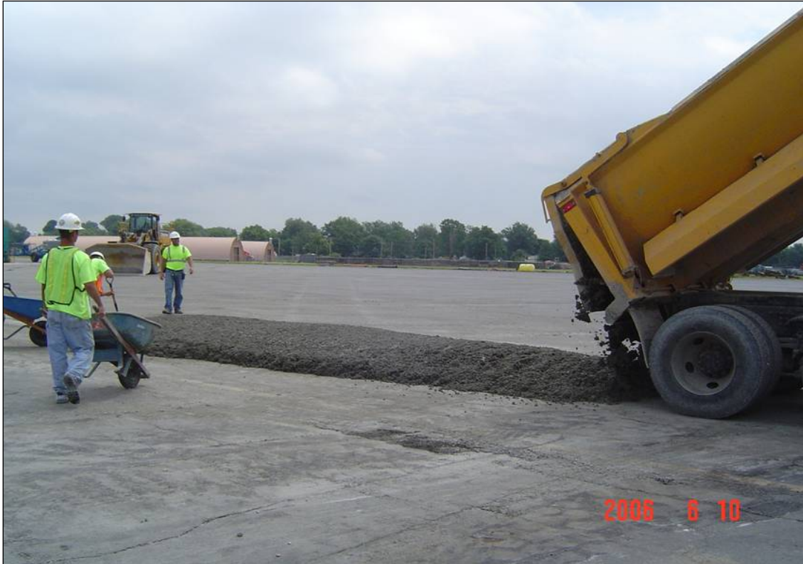
Figure 4-9 Spreading a Batch for Sampling
