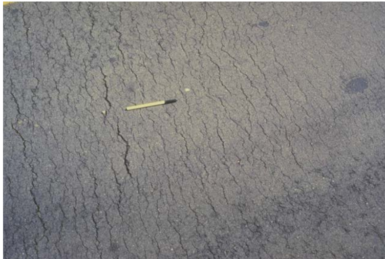
Figure 3-46 Checking Under Steel Wheel Rollers
