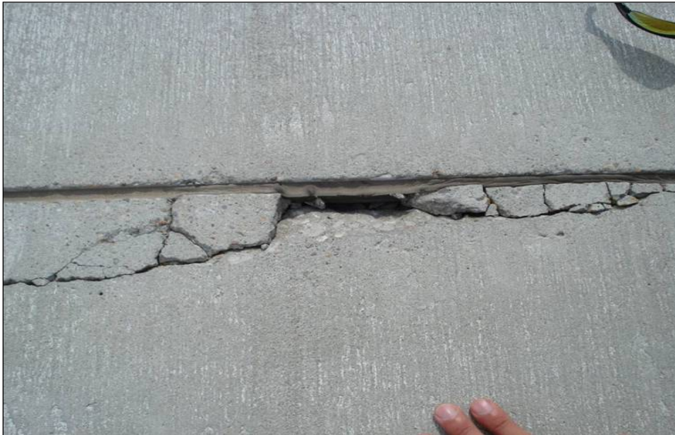
Figure 4-160 Spalls along Joint Line
