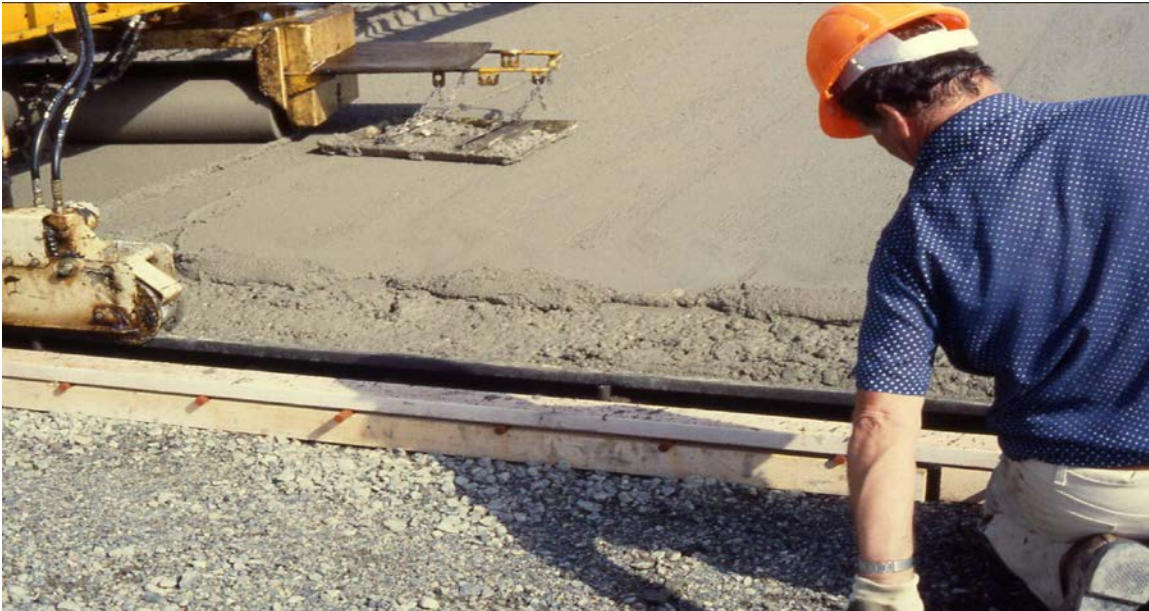
Figure 4-93 Excess Paste on Surface
