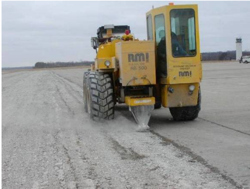
Figure 4-32 Resonant Pavement Demolition
