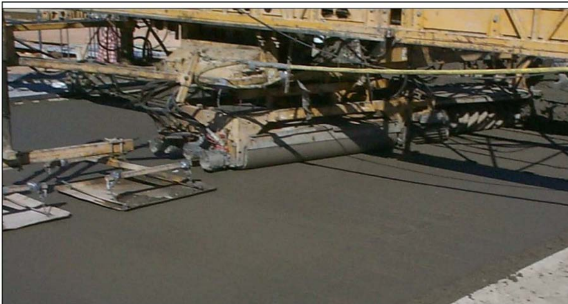
Figure 4-103 Float Pans Behind Truss-Mounted Paver
