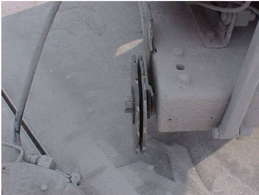
Figure 4-148 Blades used to Chamfer Joint Reservoirs
