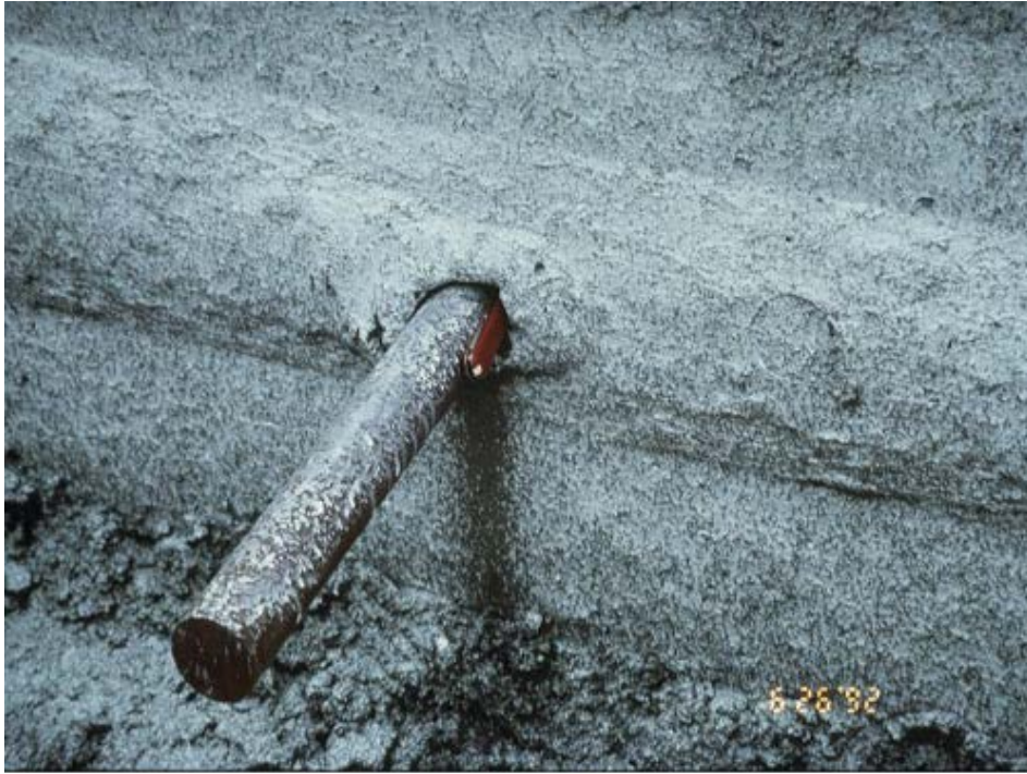
Figure 4-54 Voids around an Inserted Dowel
