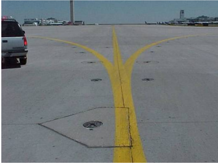
Figure 4-135 Drainage Structure – Joint Lines not matched and Random Cracking
