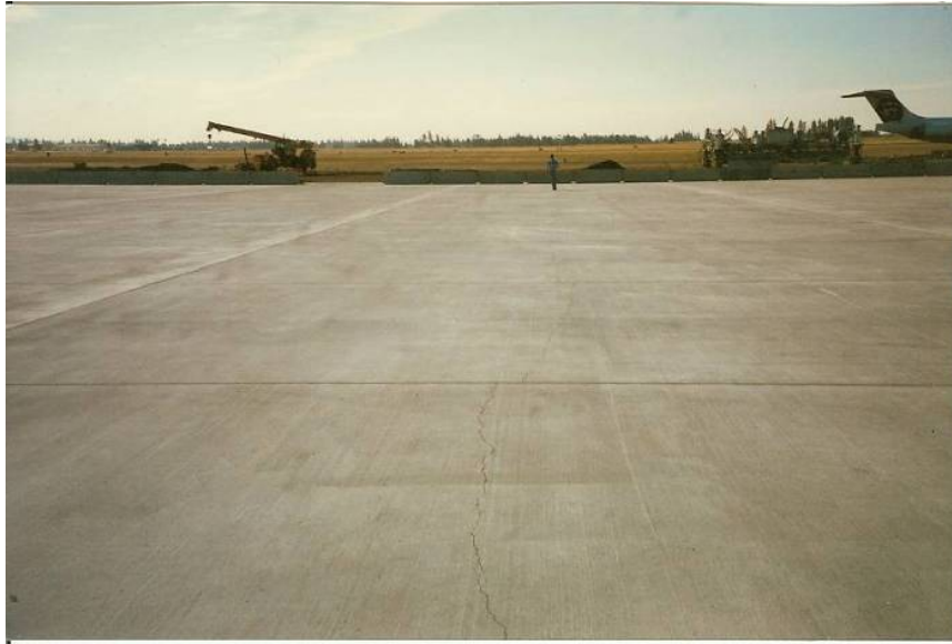
Figure 4-127 Mid-panel Cracking
