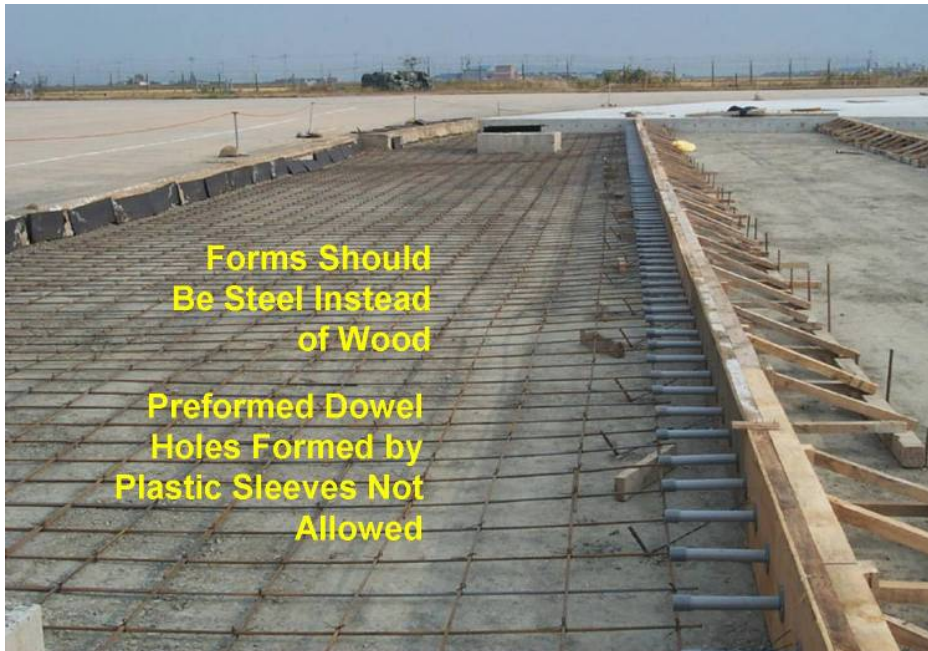
Figure 4-52 Plastic Sleeves on Wood Forms
