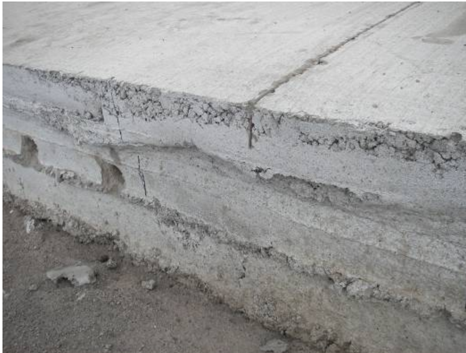
Figure 4-130 Poor Quality Thickened-Edge Joint Construction
