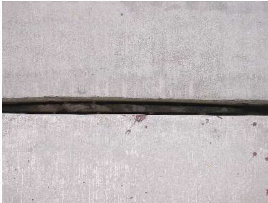
Figure 4-147 Non-Uniform Joint Cut Width
