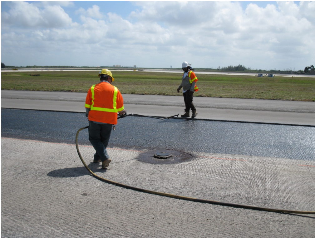
Figure 3-24 Application of Tack Coat with Hand Sprayer
