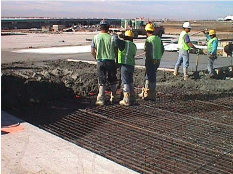
Figure 4-37 Workers Standing on Reinforcement Steel during Concrete Placement
