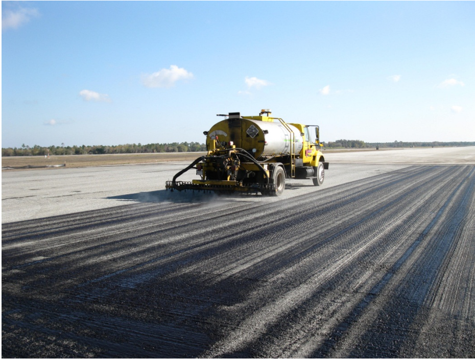
Figure 3-23 Excess amount of Tack Coat
