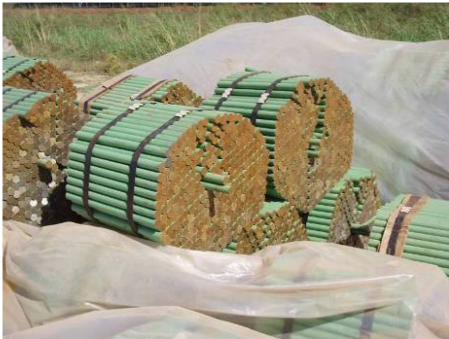
Figure 4-44 Dowels at Contraction Joints
