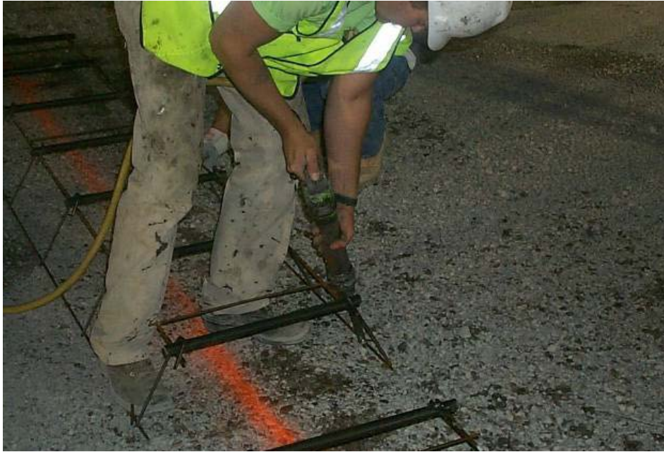
Figure 4-47 Securing Dowel Baskets
