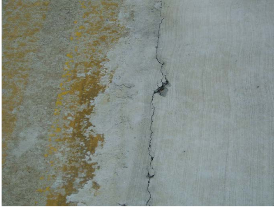
Figure 4-147 Non-Uniform Joint Cut Width
