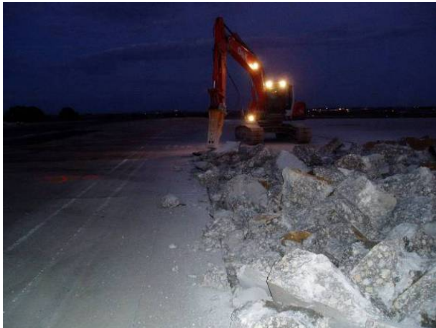
Figure 4-29 Demolition With No Protection of Adjacent Concrete
