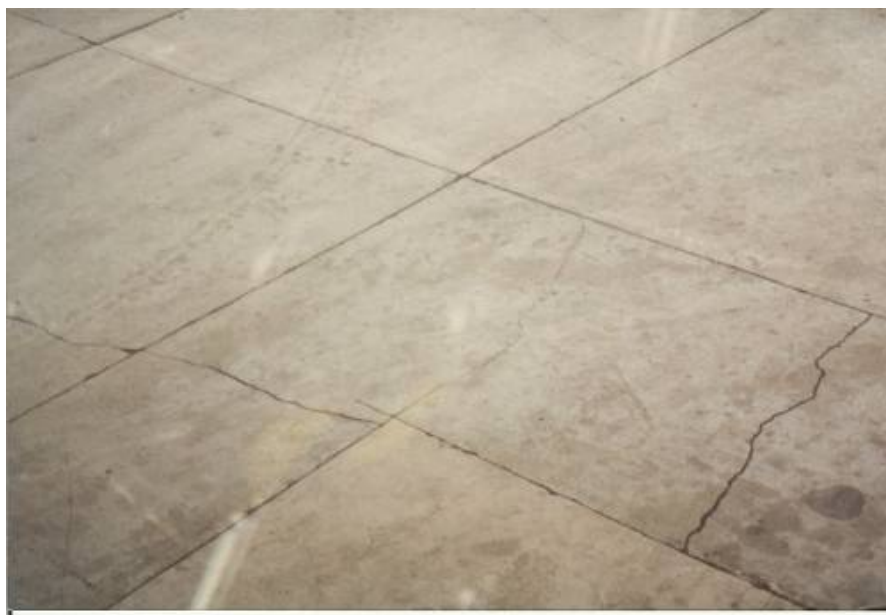
Figure 4-132 Cracks Induced by Partial Panel Replacement
