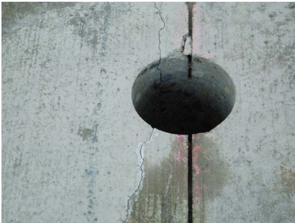
Figure 4-145 Core to Verify Depth of Crack
