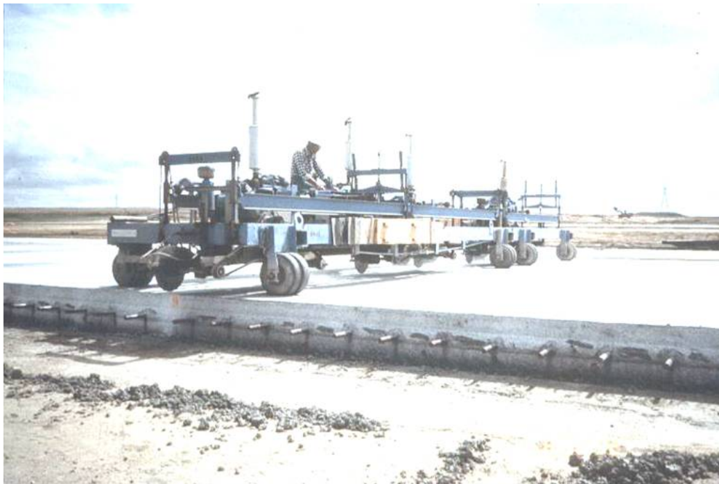
Figure 4-142 Saw Cutting Machine With Multiple Blades
