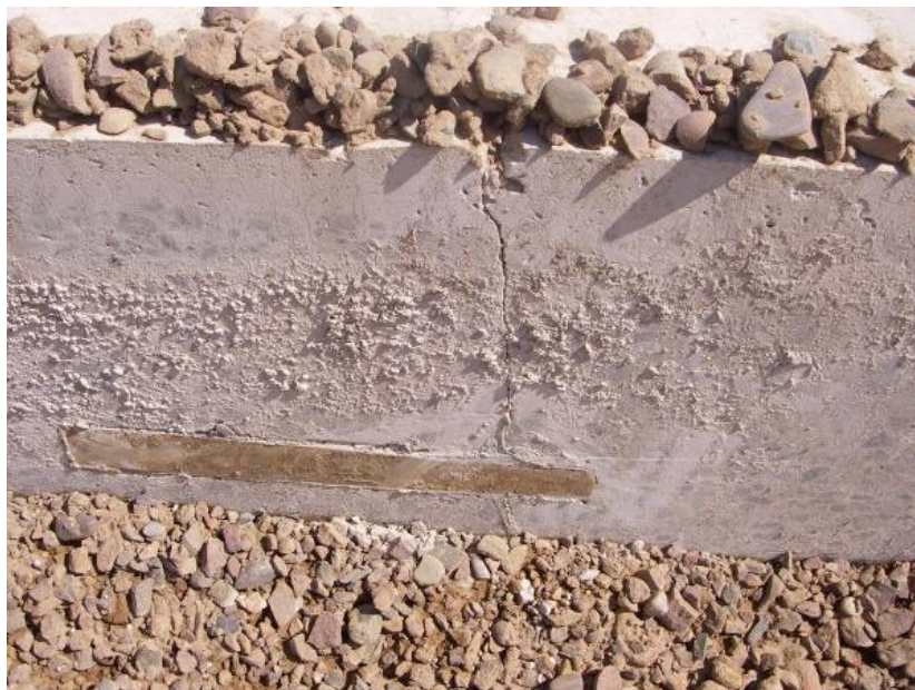
Figure 4-50 Misaligned Contract Joint Dowels
